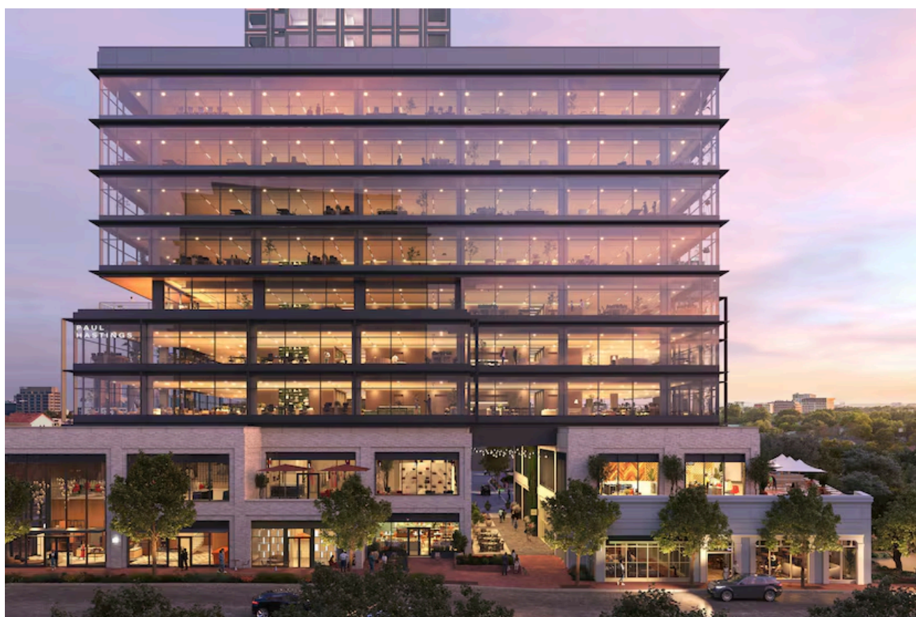
Global law firm Paul Hastings LLP has signed a long-term 37,000-square-foot pre-lease at BDT & MSD Partners, Trammell Crow Company, The Retail Connection and Highland Park Village Associates' Knox Street development. (Courtesy of Trammell Crow Company)
